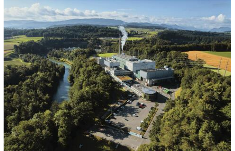
solid waste and sludge incineration plant in Posieux/Hautrive FR
